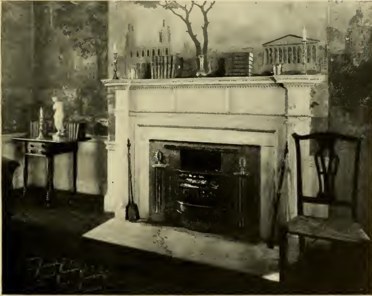
PLATE IV. — Hallway, Cabot Low House, 1748; Fireplace, Oliver House.
